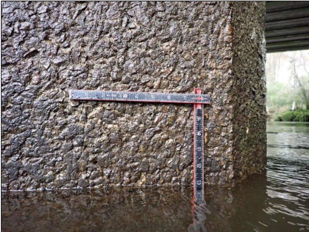
Photo 8: Typical Concrete Condition at Waterline, Bent 6, Column 3 Shown
