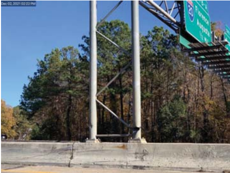
Photo #: 1 Caption: Overhead sign at west end of bridge, impact damage area with tear on metal (base of both poles next to EBL's of I-26 shown)
