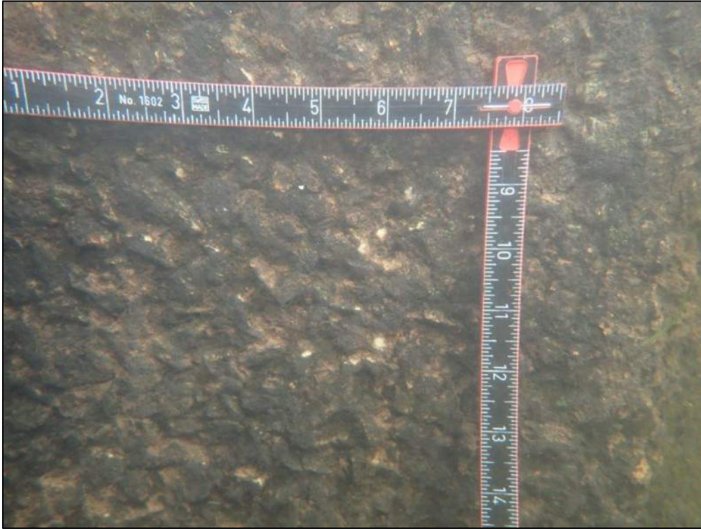
Photo 9: Typical Concrete Condition Below Waterline, Bent 6, Column 3 Shown
